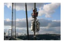
self-driving up to 120 mm cable diameter
