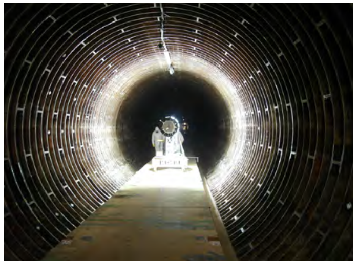
Inspection of the tunnel under rehabilitation
