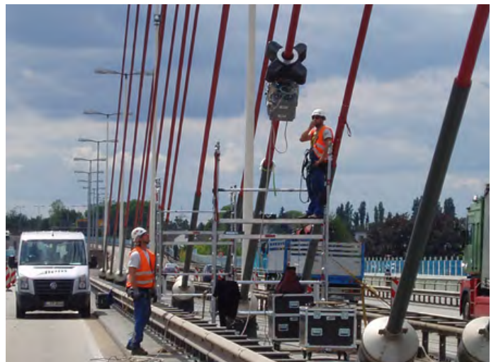
Neuwied Bridge: erection time approx. 20 minutes
