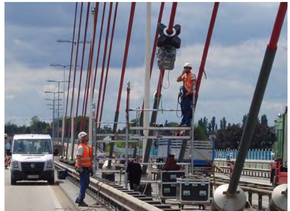
Neuwied Bridge: erection time approx. 20 minutes
