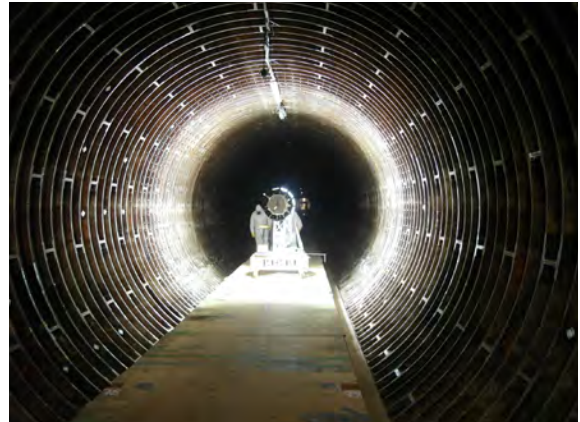
Inspection of the tunnel under rehabilitation
