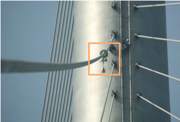
Cable inspection on Stonecutters Bridge, Hong Kong
