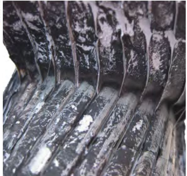
Tape peeled off from cable surface after wrapping
