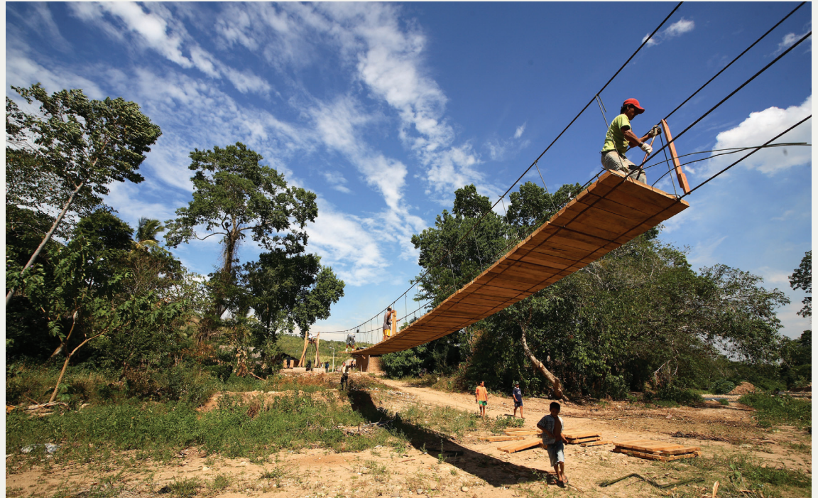
Above: Construction of the wooden footbridge deck. Below right: The bridge towers being erected
