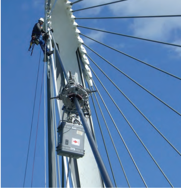
Left: Wrapping in progress; the operative above is working at the end of the cable. Above: View of the structure with its twin decks and cable planes.
