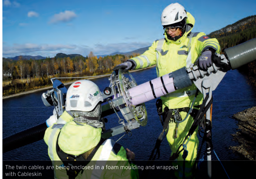
Twin cables are the main support – at the saddles there are discontinuities in the outer wires
